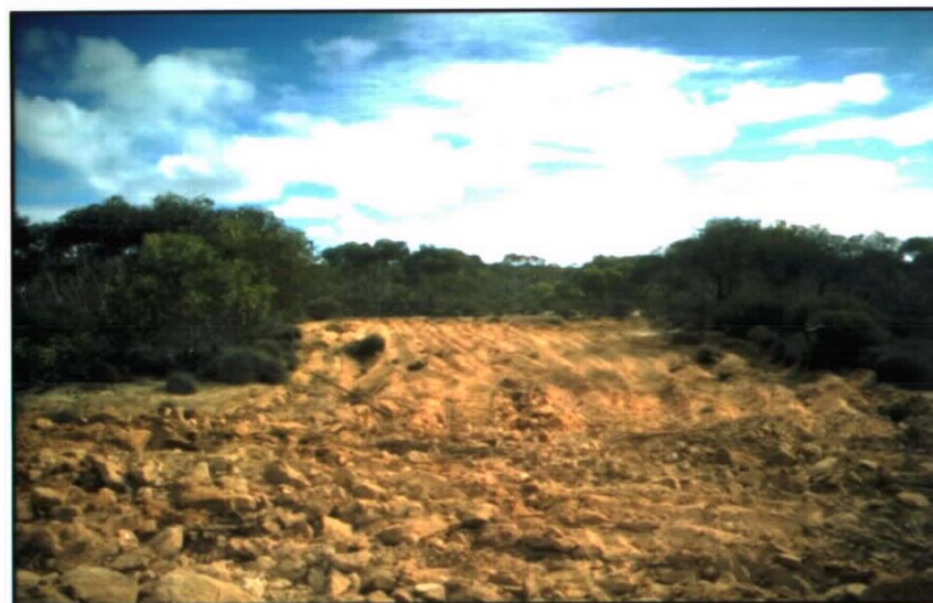
Plate 6. Borrow pit after ripping. (Photo 43718)
