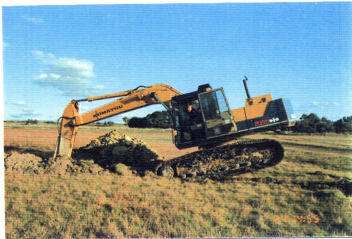
PLATE 8: Pit 11 - Refusal of excavator on strong calcarenite.
