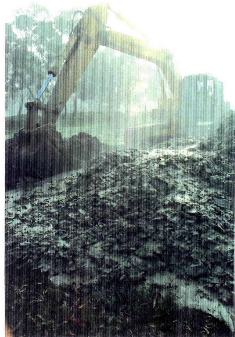
PLATE 4: Pit 9 - Spoil- Note granular, blocky nature; wet, sloppy digging conditions. Photo No. 40286
