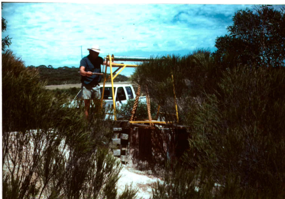
Plate 1 Mount Hope Kaolin Deposit - Site of shaft sunk to 21m in 1973 to obtain a 40 tonne bulk sample.
