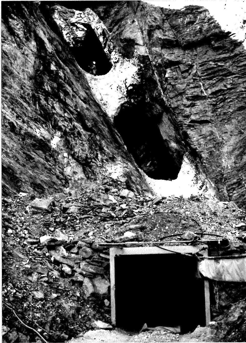
Plate 2. Decline portal to the Oraparinna Barite Mine.
