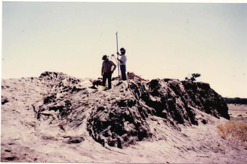
PLATE 3. Hand auger drilling of tailings stockpile at old Mongolata Battery site. Slide No. 36617
