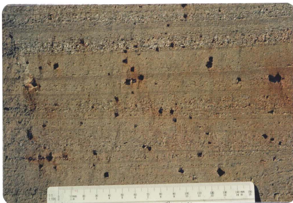
PLATE 7. GLADSTONE GAOL - CUBES OF BROWN LIMONITE AFTER PYRITE IN WALL. Closeup of graded bedding in sandstone and random cubes of pyrite altered to red brown limonite. January 1984. Slide No. 36009
