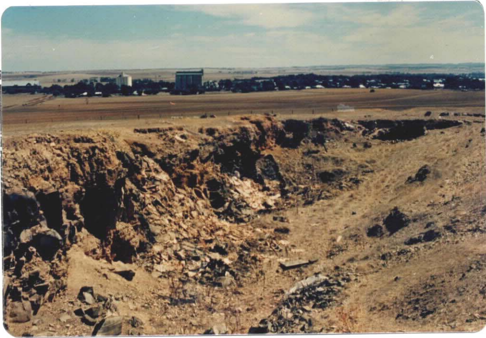
PLATE 1. NO. 2 QUARRY - VIEW NORTH WEST Face at left to 8 m high, partly obscured by rubbish. Floor overgrown. Gladstone township in background. No. 1 Quarry not visible but in front of houses and behind tree at mid centre right. February 1984. Slide No. 36003
