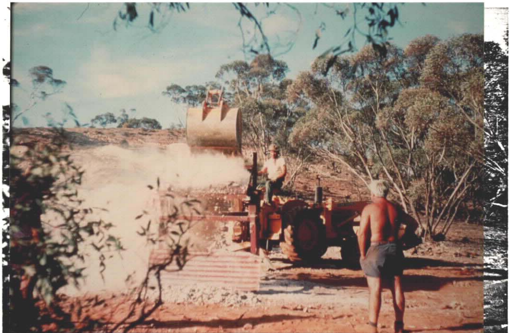
PLATE 6. Screening bulk sample from No. 2 Open Cut at North Medora prior to treatment at Peterborough State Battery.
