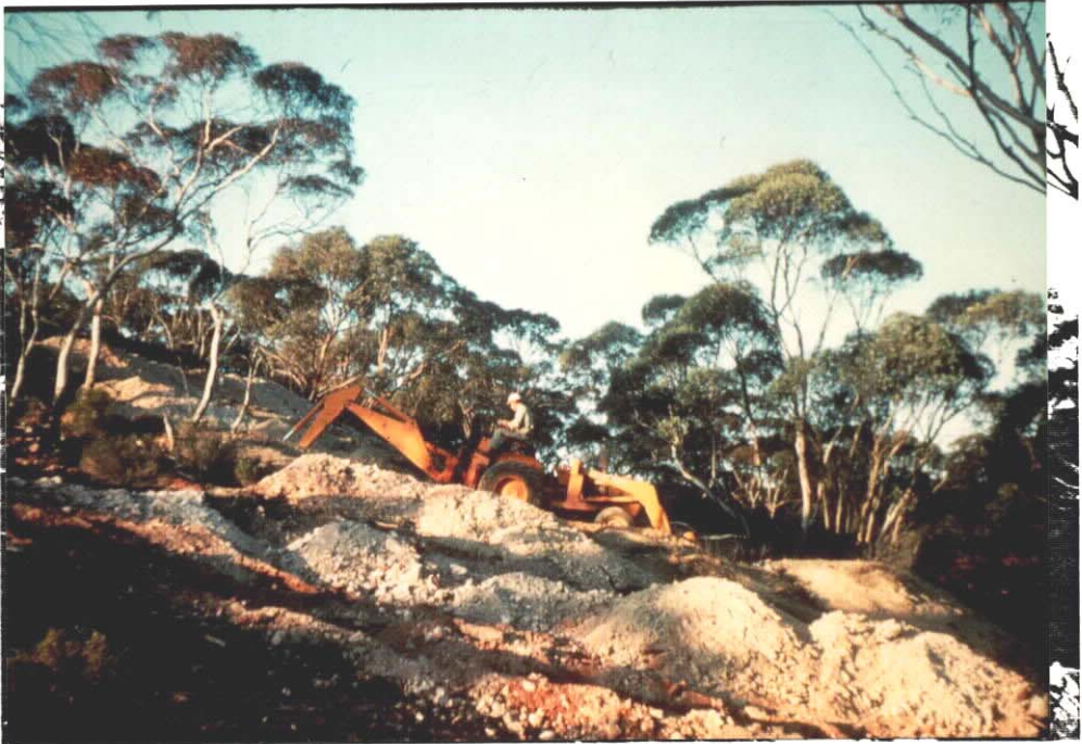
PLATE 5. Excavating Trenches for Sampling at North Medora.
