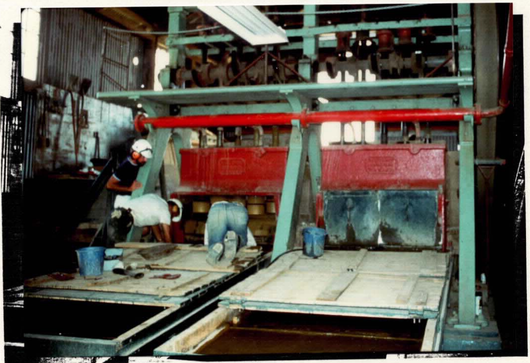
PLATE 13. Cleaning and Scraping the plates at Peterborough State Battery. Slide No. 36067
