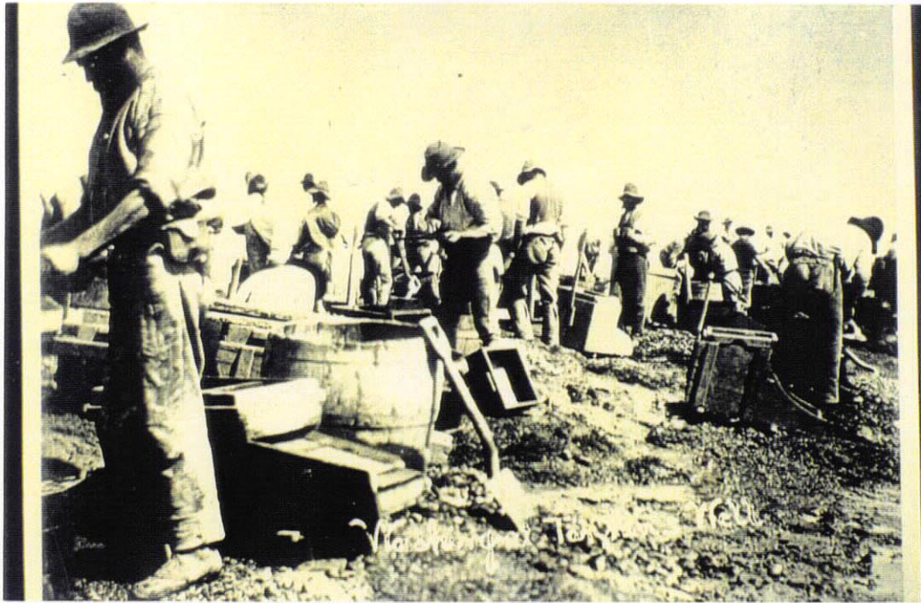
PLATE 13. Cradles and Rockers in use at Tonkin's Well, Teetulpa, 1886. Slide No. 35291
