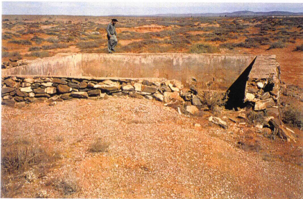
PLATE 14. Remains of Cement Rendered Stone Tank at Tonkin's Well, 1986. Slide No. 35292
