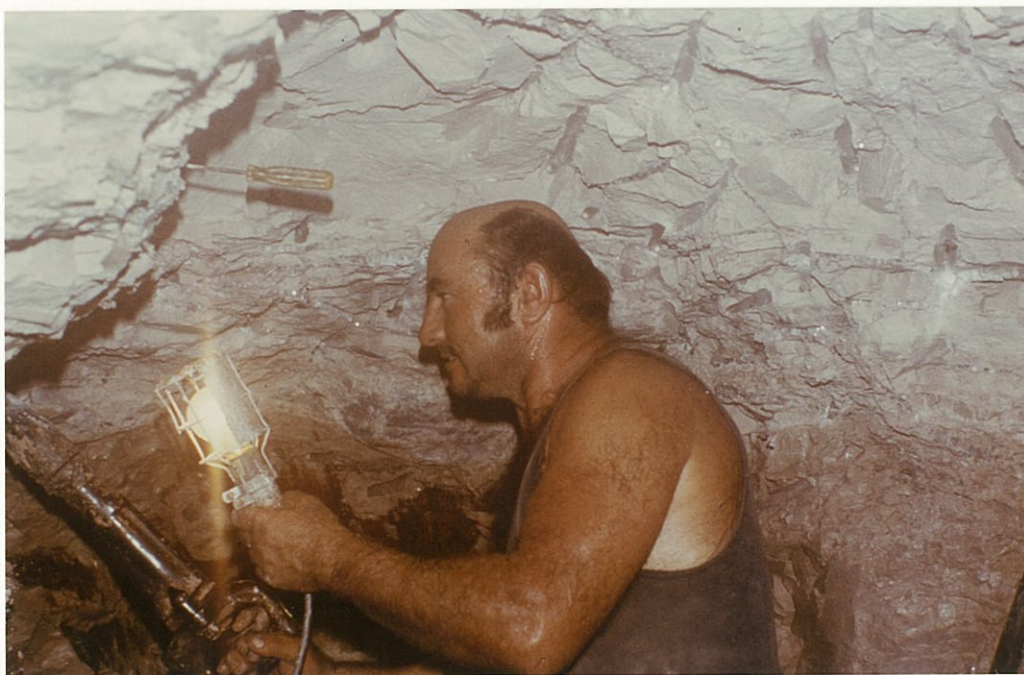
PLATE 12 - Driving opal level, Subsidised Shaft 17, Andamooka June 1976. 'Opal level' marked by boulders at contact of white 'kopi' above and dark 'mud' below. (slide 13772)
