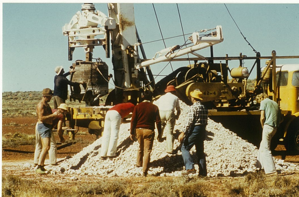
PLATE 7 - Calweld drill, Andamooka 1976. White 'kopi' being inspected for signs of 'opal level' at Subsidised Shaft 6. (slide 13756)
