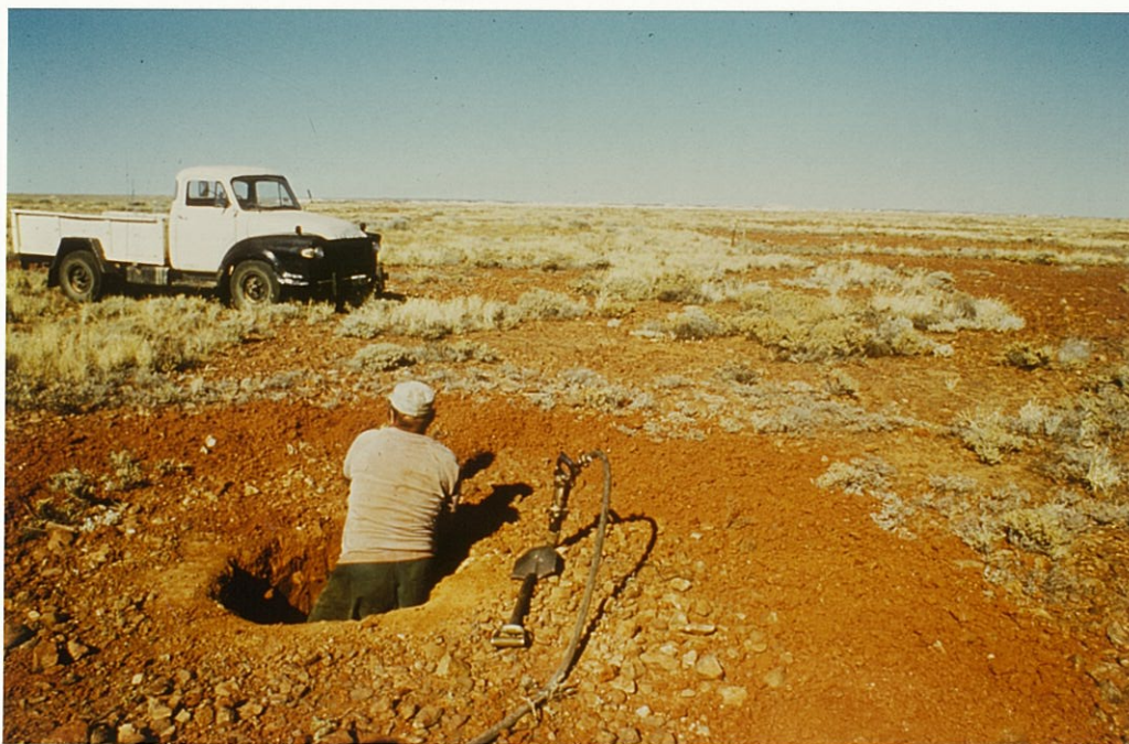
PLATE 8 - Collaring Subsidised Shaft 2, Andamooka May 1976. The first shaft to be started in the exploration program. Jackpick and compressor being used. (slide 13770)
