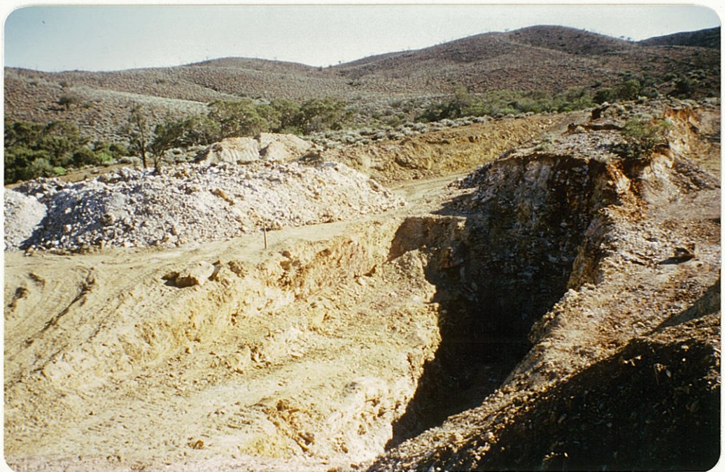
PLATE 4. Nilpena 2A Lode opencut. View northeast over open cut showing footwall and hanging wall platforms, deep slots on hanging wall and on the lode. Stockpile of barite centre left. Bitter Springs Creek is in the left background. (October 1980). SLIDE NO. 23145.
