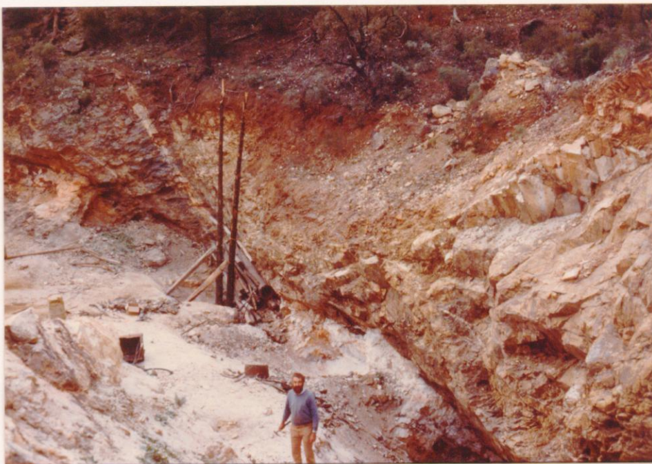
PLATE 2. McRae Deposits - No. 1 Lode. View westwards of western end of main workings, 670 m bench. Shaft No. 1 marked by posts. Hanging wall, massive quartzite and sandstone, footwall left foreground. Barite lode bifurcates at western end. (June, 1979) Neg. NO. 32486.
