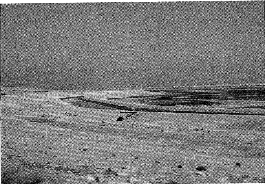
Canal constructed across Lisan Peninsula to connect shallow southern arm to main deep sector of Dead Sea
