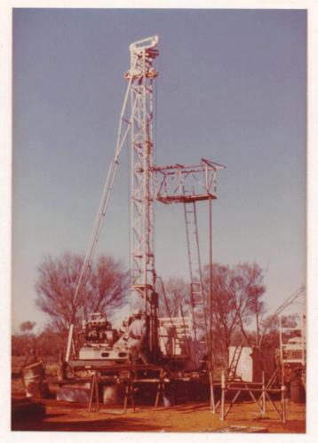
PLATE 1 Mindrill 10L diamond drill rig onsite at Byilkaoora 1. (Transparency No. 14751; Neg. No. 30876).
