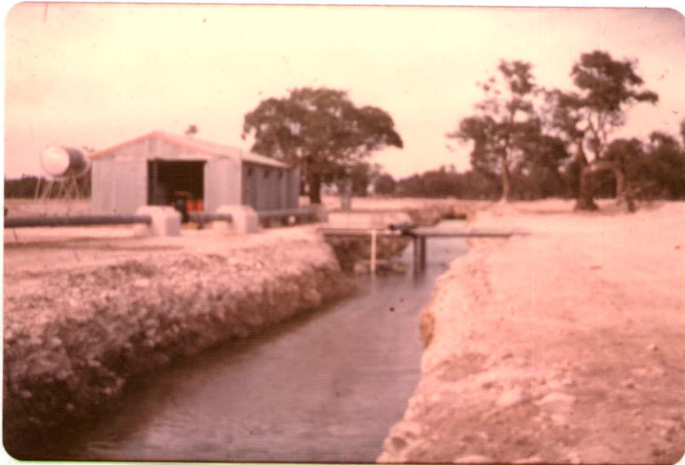
Polda Basin, Eyre Peninsula. Pumping station and trench with exposed water table, 1962. Trench is approximately 60 metres in length and is now covered.
