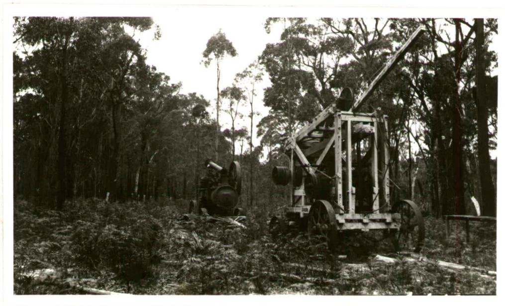
Cable tool drilling plant, operated by steam engine (background) about 1912.
