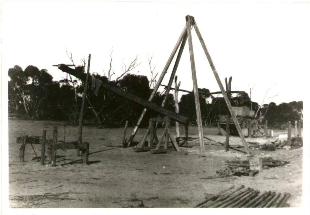
Hand drilling plant used for test wells, hundred of Perlubie, near Wirrulla, 1912.
