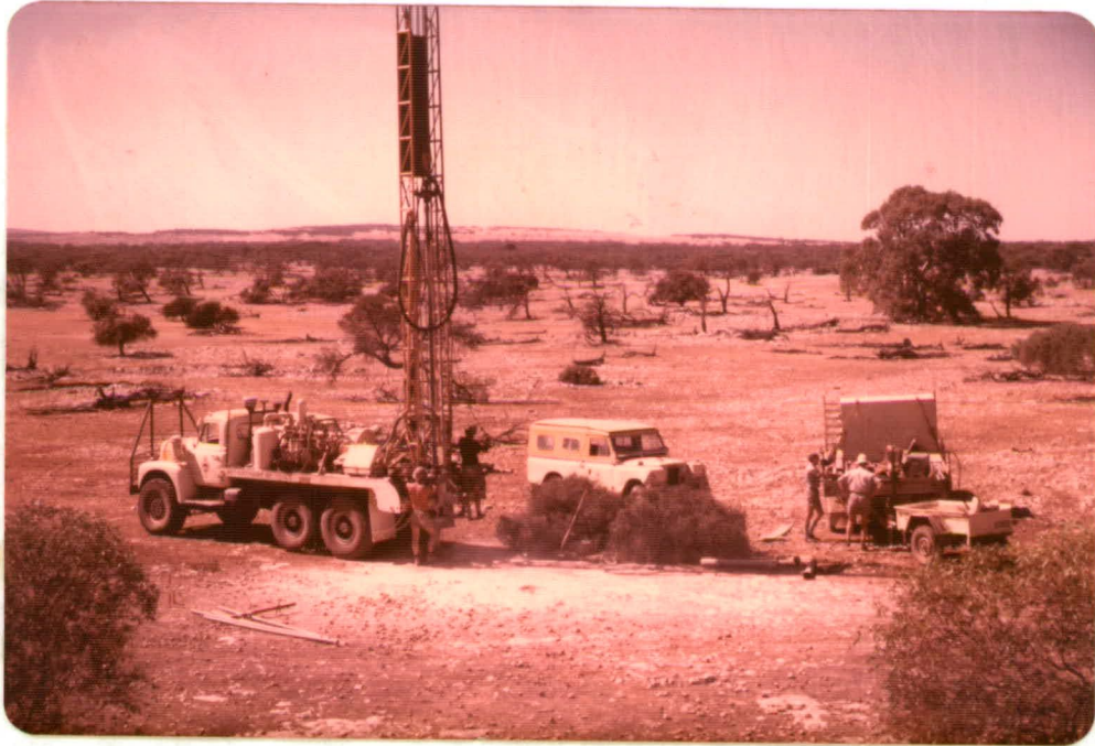
Mayhew rotary drilling plant County Musgrave, Eyre Peninsula, 1968.
