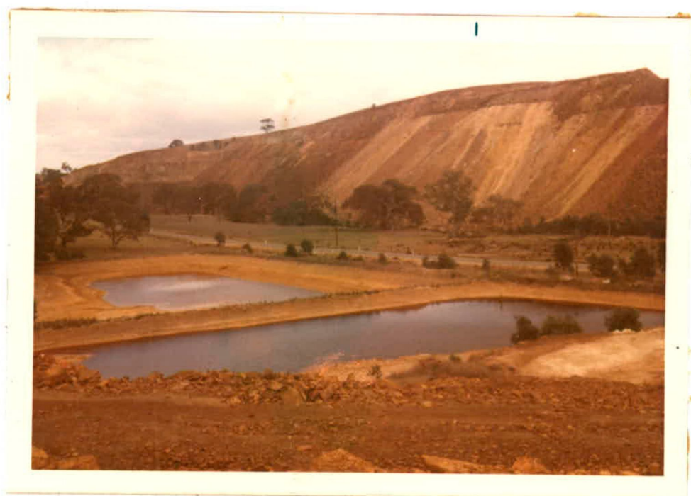
PLATE 10: Holding ponds for AMD at base tailings dam. Facing south, the Dawesley runs along base of coarse waste dump on right.
