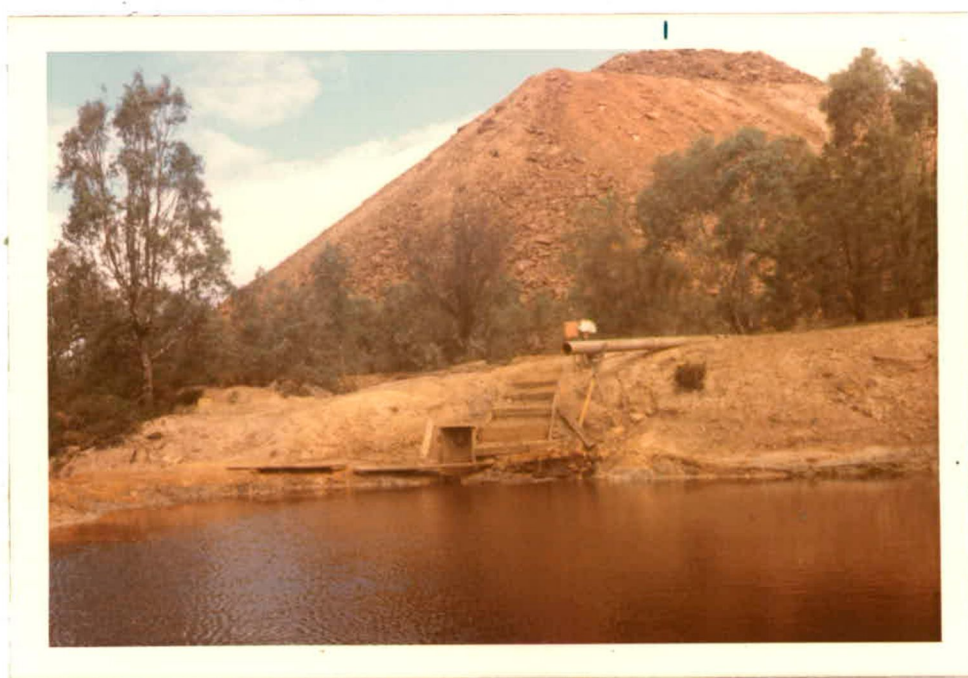
PLATE 11: Holding pond for AMD from northern quarry. QSB enters through pipe at centre. The Dawesley, out of picture on the left, runs adjacent to the pond.
