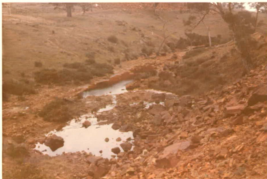
PLATE 7: Seepage (QSD) entering Dawesley Creek in southern mine area from former creek bed below waste material at bottom right.
