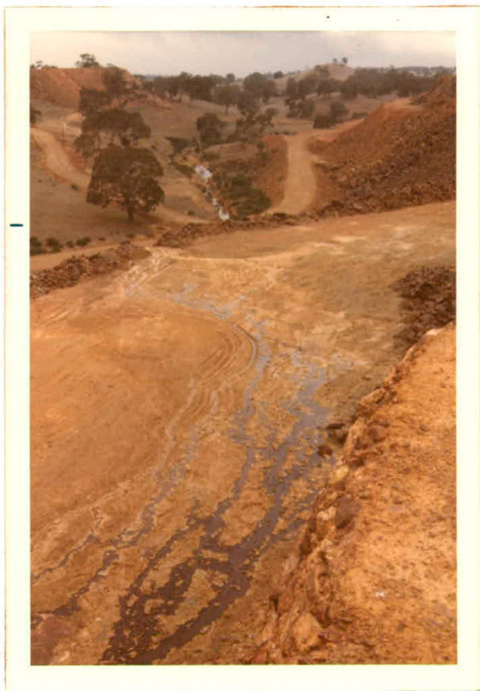
PLATE 1: Seepage (QSC) running along quarry bench in foreground; eventually reaching Dawesley Creek in background
