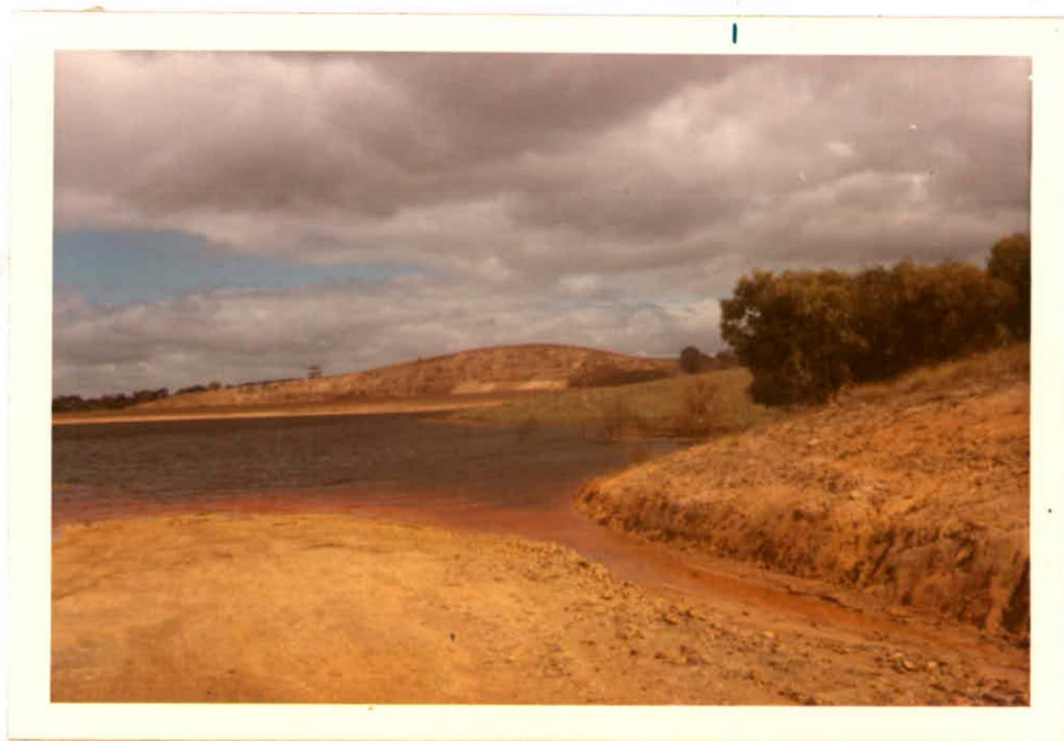
PLATE 9: Upper holding pond for AMD on tailings dam showing red-blue coloration of the oxidised drainage and quarry face in background.
