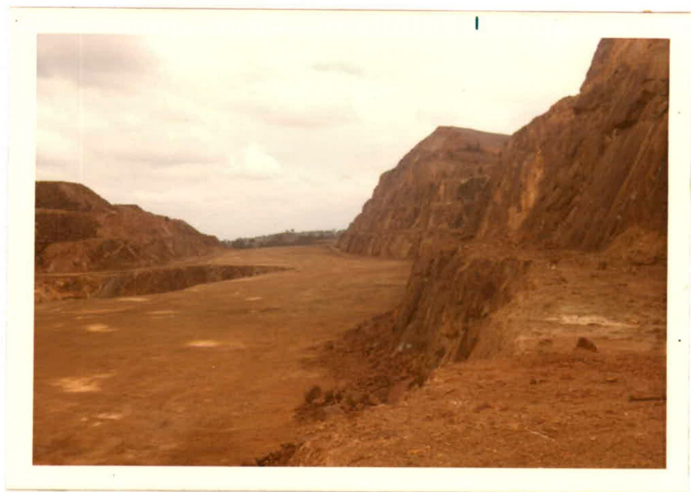
PLATE 3: Open-cut quarry facing south from central position; benches to right and coarse waste dumps to left.
