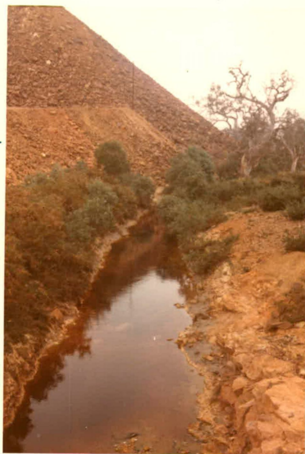
PLATE 6: Dawesley Creek in southern mine area. Channel cut to allow passage of creek water. Waste dump on left covering old creek bed.
