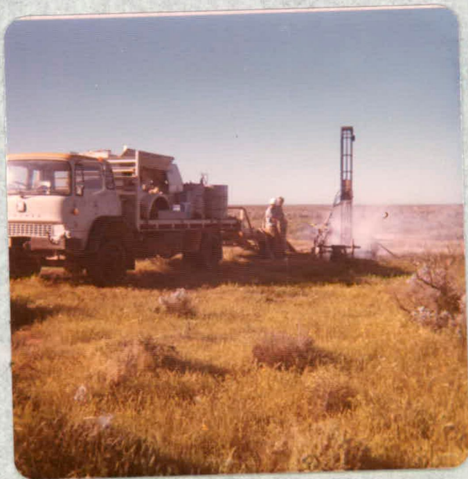
Photograph 2. Halco Rotary Percussion Drilling Rig with compressor on the truck.
