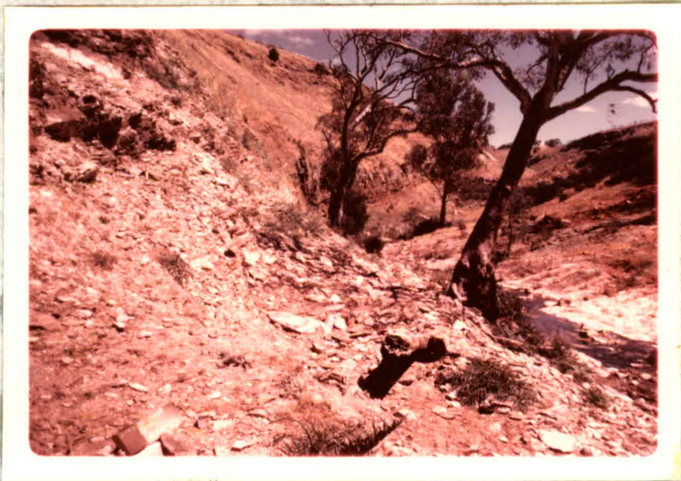
Plate 1. View along Outlet Duct Alignment taken from proposed Outlet Tower Site.
