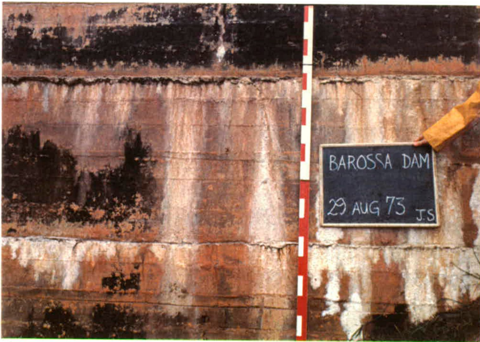
3. Closeup of "day plane" crack
