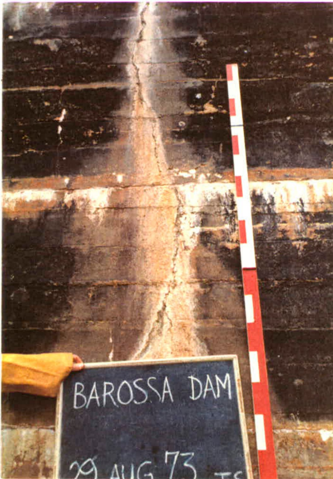
2. Closeup of vertical crack.
