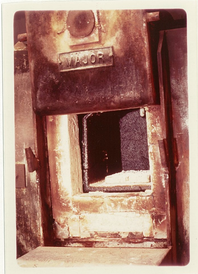
22109 Lightweight Aggregate Project. Oil-fired Muffle Kiln. AMDEL.
