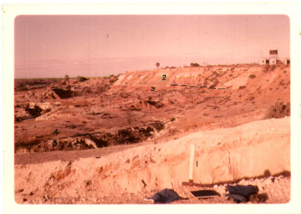
Chowilla Damsite. Left or S.E. abutment: (1) Loveday Soil. (2) Upper Member of Blanchetown Clay over (3), Lower Member. (4) Sandstone cap over (5), Parilla Sand.
