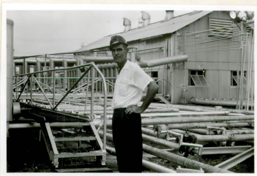
Fig. 81 Hot-water and molten sulphur lines, Newgulf.
