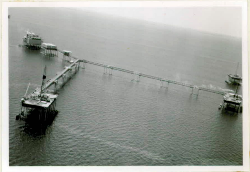
Fig. 92 Grand Isle Mine (Freeport Sulphur Co.). Power Station, living quarters and heliport on distant arm. Production wells and drilling platform at left and right. Bleed Well at distant right.
