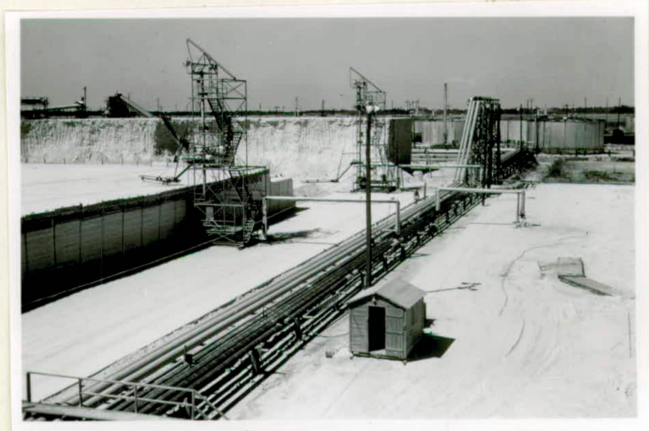
Fig. 83 Sulphur lines and vats, Port Sulphur (Freeport Sulphur Co.)
