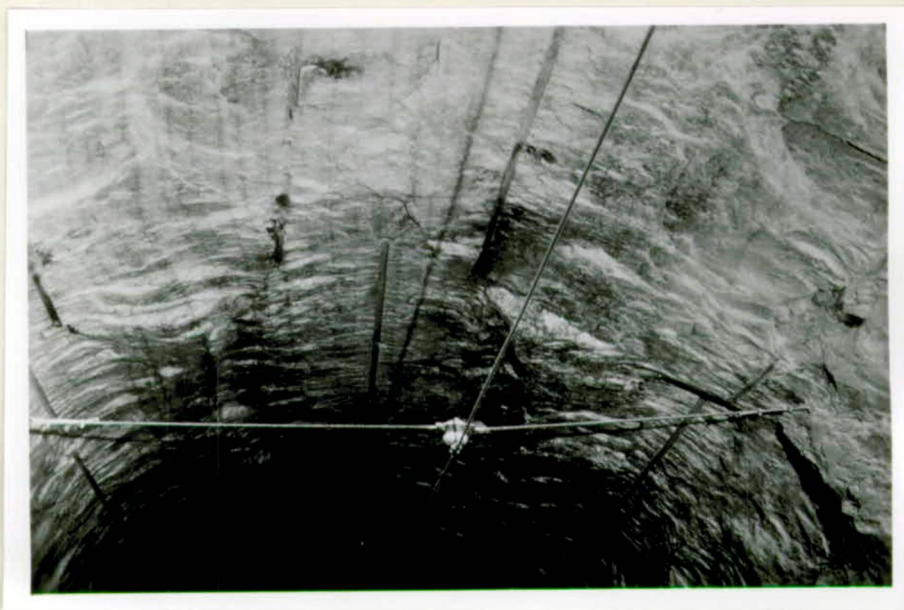
Fig. 16 7 Leinne salt enclosing Ronnenberg potash seam, Ronnenberg. Potash seam exposed on right side of roof of drive above electric cable. (R. Russell photo)
