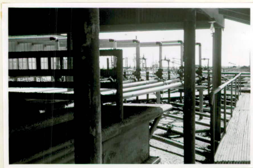
Fig. 82 Molten Sulphur collecting station. Long Point Dome, Texas (Jefferson Lake Sulphur Co.). Oil production well in right Background.
