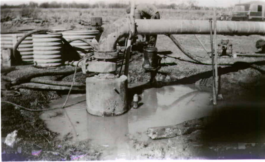
Cementing operations - reconditioning an old bore
