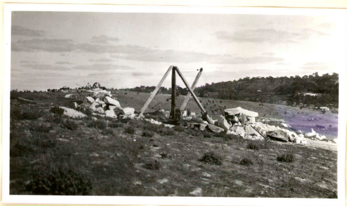
VIII. Production of dimension stone, Sec. 339, Hd. Moorooroo.
