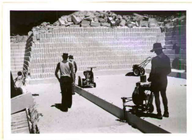
XII & XIII. Mt. Gambier limestone quarry. Dimension stone being cut directly from the face and floor of the quarry.
