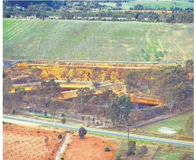
The Brukung acid leachate holding ponds (foreground) with the tailings dam wall and rehabilitated tailings dam behind, 1996. (Photo 45909)
