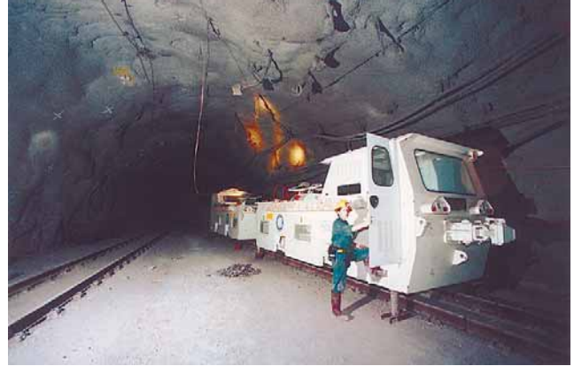
Commissioning of the 25 t locomotives and section of the track. (Photo 46508)
