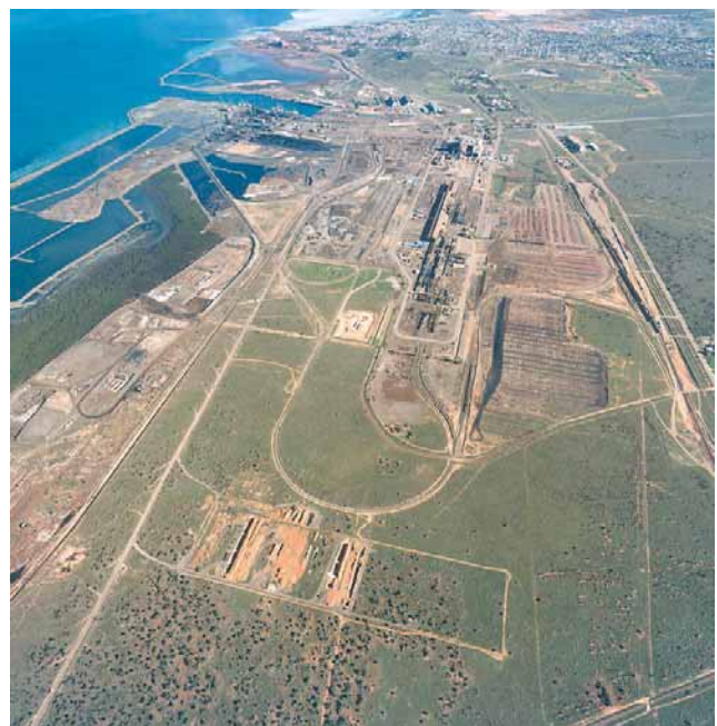
BHP Whyalla Steelworks, with the City of Whyalla in the distance. (Photo 46673)
