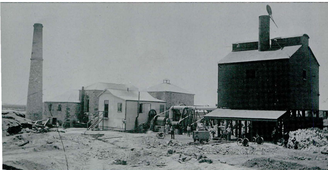
Yelta Mine, c.1905. The old stone buildings still survive and, at right, is a water-jacketted blast covered by a galvanised iron shed. The small iron building housed a blowing machine which produced the air blast. PIRSA 039658
