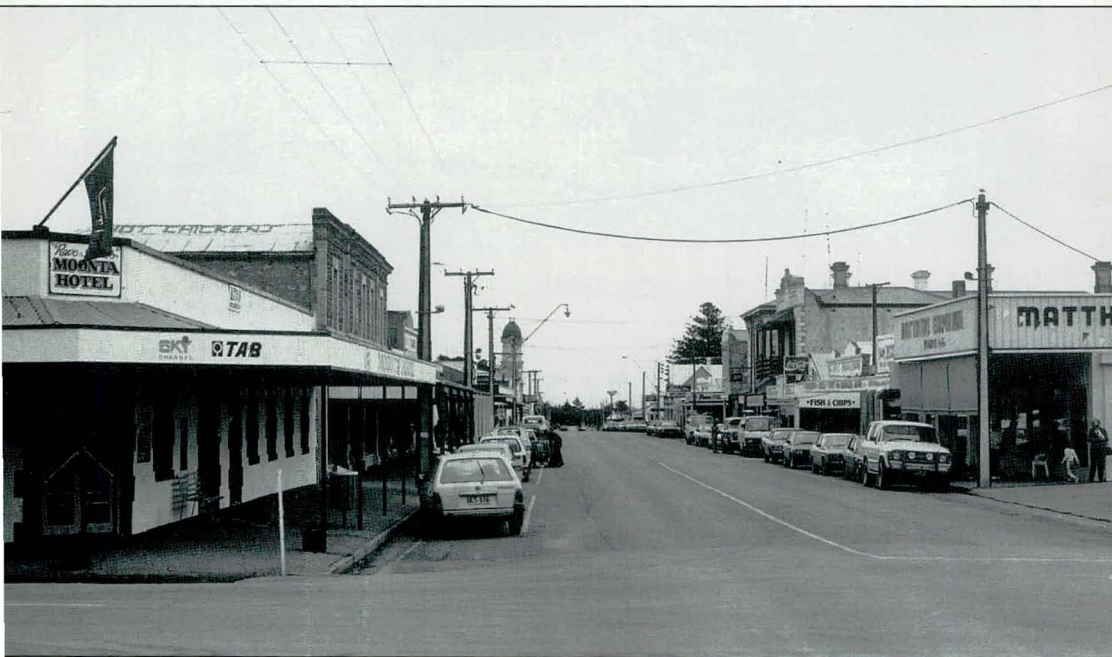
George Street looking west from Blanche Terrace. Upper: c.1895. Note the horse drawn tram. PIRSA 039682 Lower: 1990. PIRSA 039683
