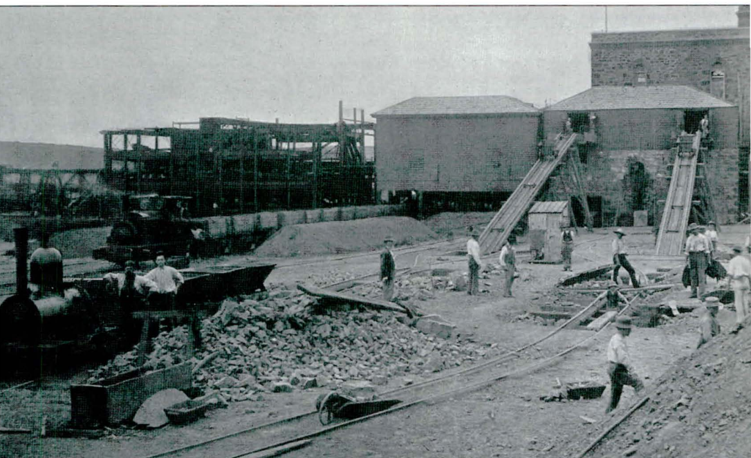
Richmans Enginehouse and concentration plant, c.1900. PIRSA 033340
