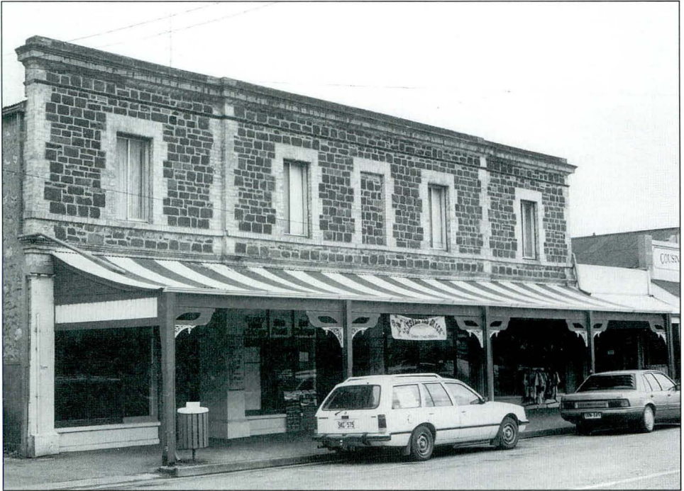
Marshall building, George Street. PIRSA 039681
