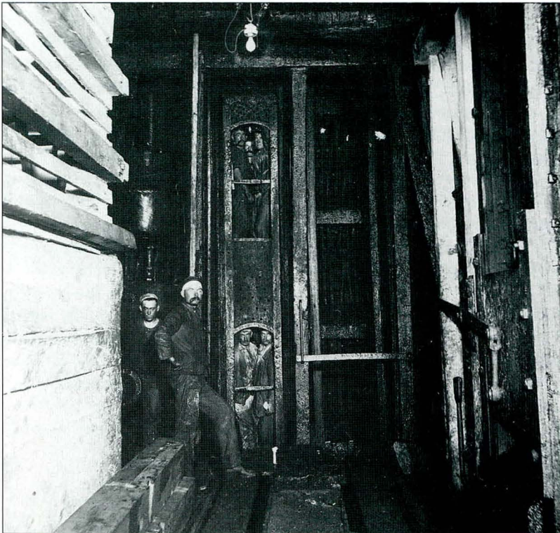
Double-decker man skip which was introduced after 1880. PIRSA 030191
