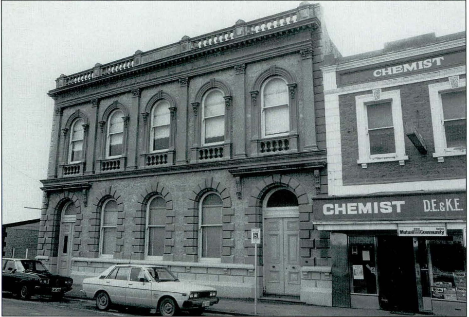
Former Union Bank, Ellen Street. PIRSA 039669
