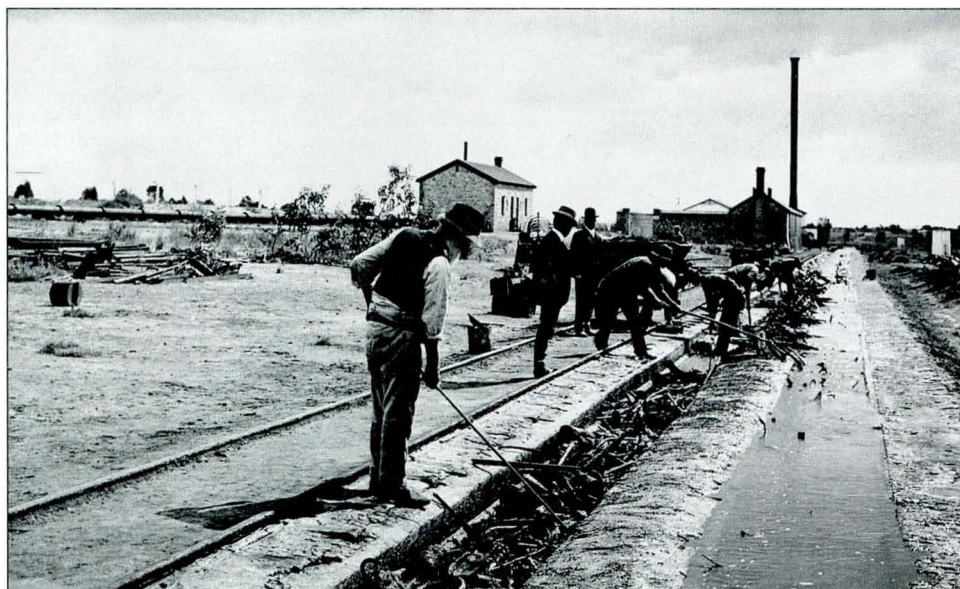
Precipitation works looking west along precipitation channels from Dry House to Pumping Station, c.1910. Men are removing scrap iron from the channels to recover the precipitated copper sludge. PIRSA N007170
