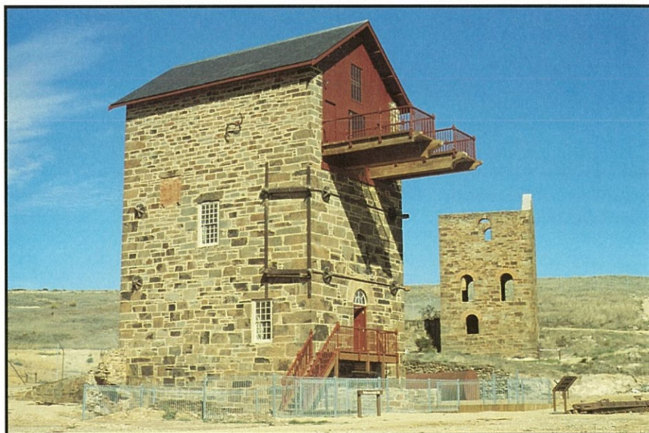
Morphetts Enginehouse after its reconstruction in 1986, with Morphetts Windinghouse in the background. (Photo no. 37803)
