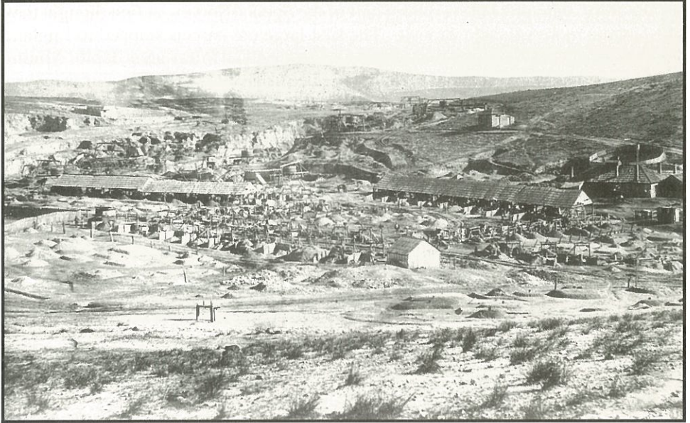
ABOVE: Ore dressing floors, c. 1865, containing numerous rows of hand-operated jiggers. (Photo no. 12975)
