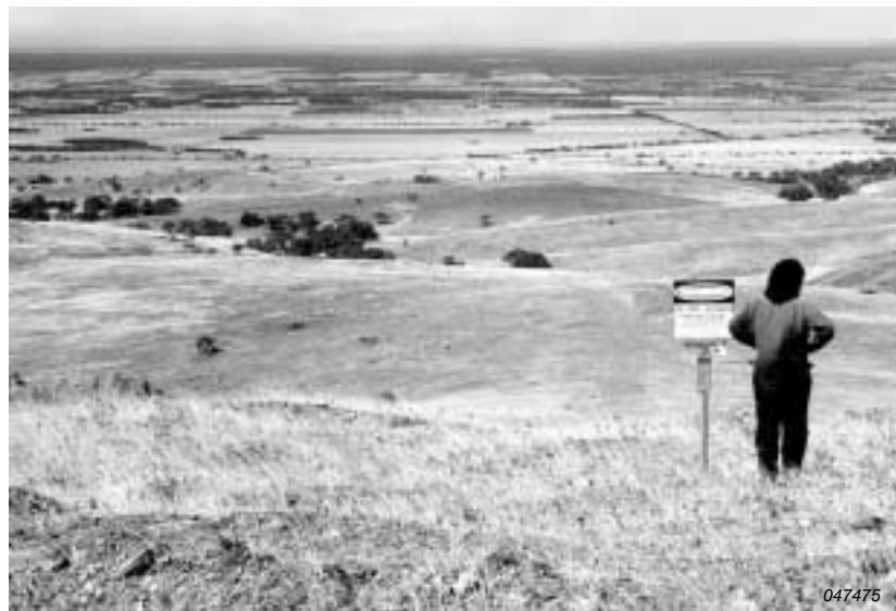
Riverland pipeline looking towards Sedan; pipeline runs downhill immediately left of the sign. Pipelines are normally buried and such warning signs and mainline valves are their only visible indicators.
