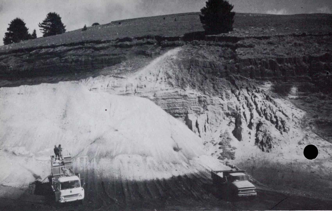
Hydromulcher at Mount Schank quarry.
