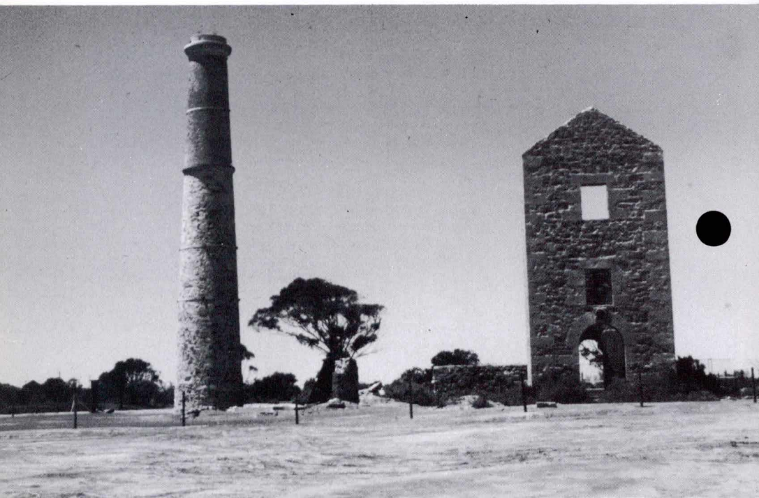
Hughes enginehouse and chimney, Moonta Mines (Neg. 34488).
