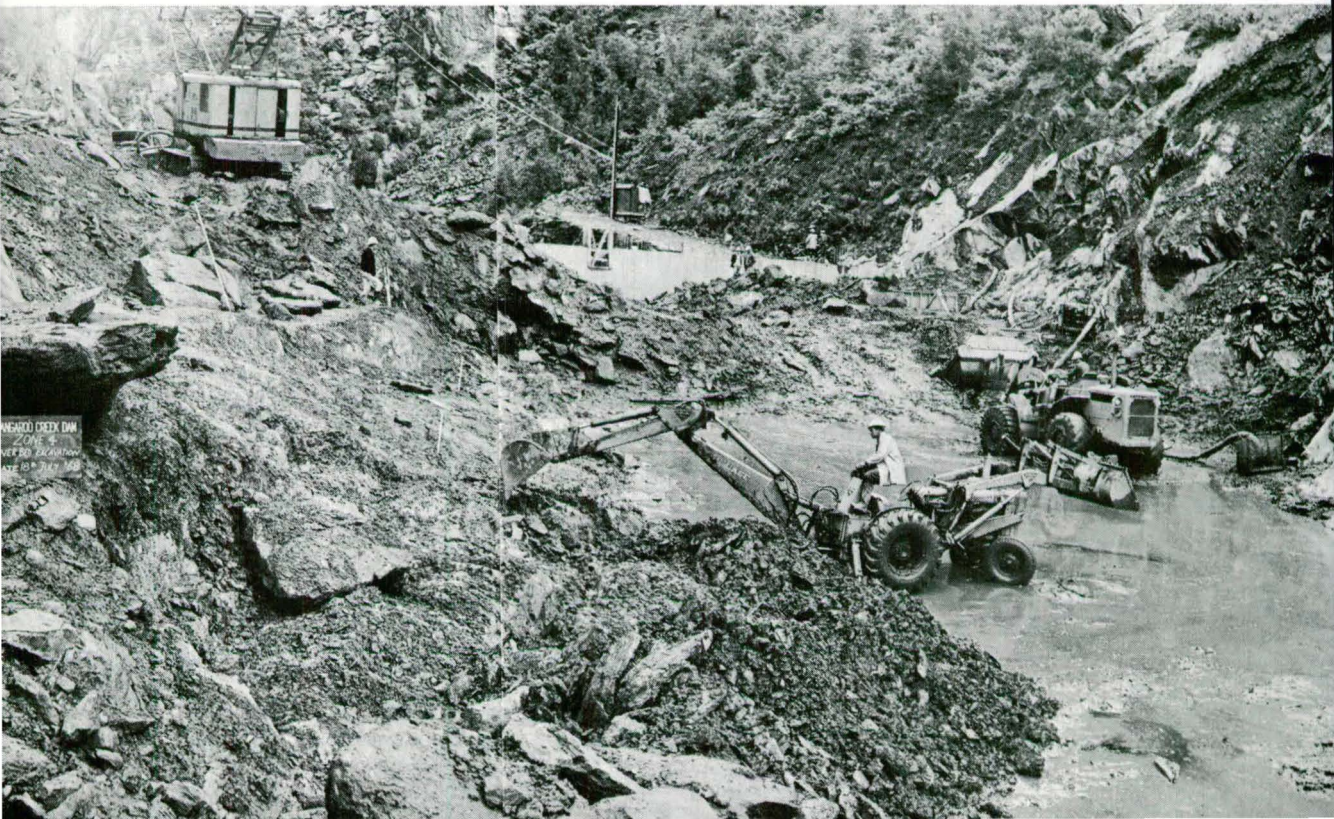
Fig. 23. Foundation clean-up in downstream part of river bed.
