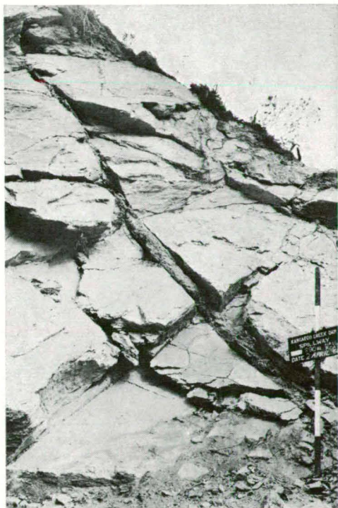
Fig. 17. Seam of infilled clay in a Set (2) joint which forms one side of a semi-detached wedge of rock.
