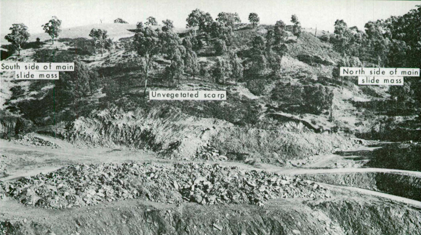
Fig. 89. Large landslide at the head of the gully to the south of the dam. The disposal area in the foreground is mainly above full supply level and supports the toe of the slide.
