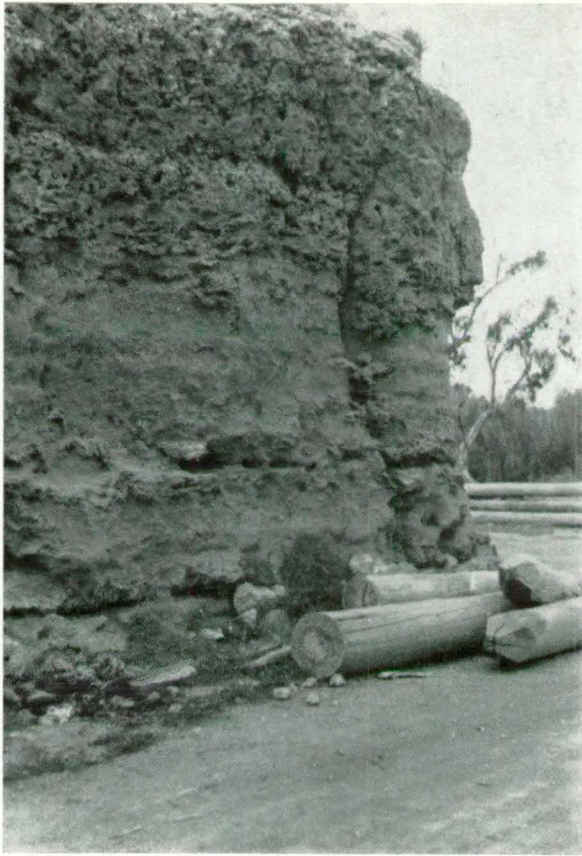
FIG. 13—MANNUM FORMATION AS EXPOSED BEFORE LEVELLING Mannum pumping station
