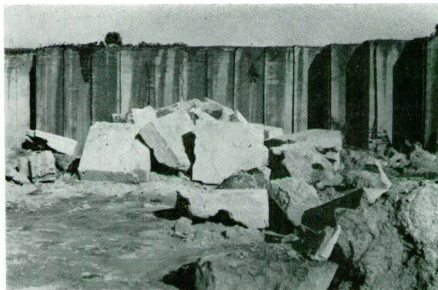
FIG. 8—SOLUTION CAVITIES IN GAMBIER LIMESTONE Kain and Shelton Quarry
