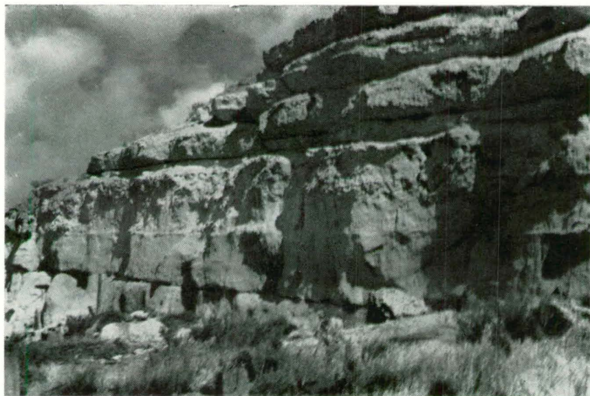
FIG. 24—MORGAN LIMESTONE Morgan railway station yard
