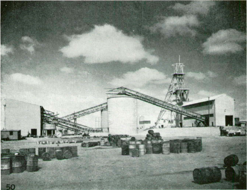
FIG. 50—RADIUM HILL MINE Showing headframe, crusher-station (at right), storage bins, and concentrator
