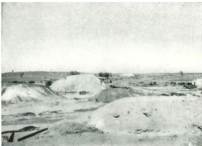
FIG. 75—GENERAL VIEW OF THE MUTOOROO MINING AREA— LOOKING SOUTH FROM THE OLD MAIN SHAFT The line of lode is marked by dumps extending into the background— Leaching-vats and precipitation canals at right
